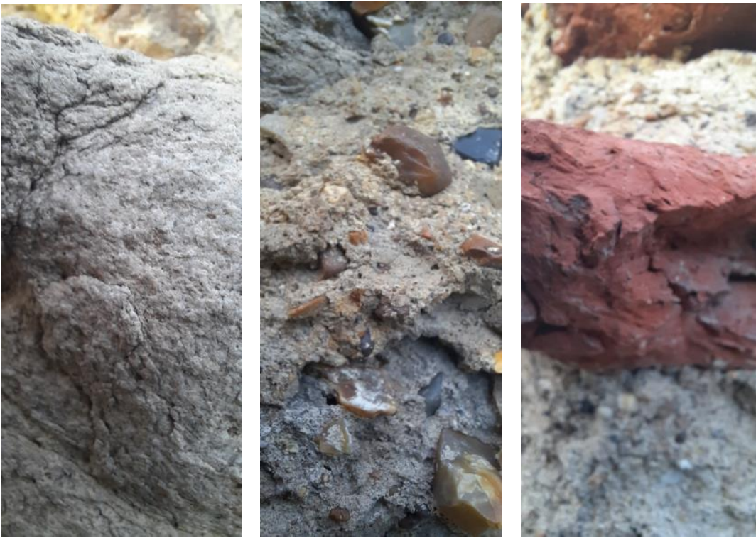
Figure 11: © Parts of the Tower Hill wall from left to right; Kentish ragstone building block, Roman cement, Roman tile.
